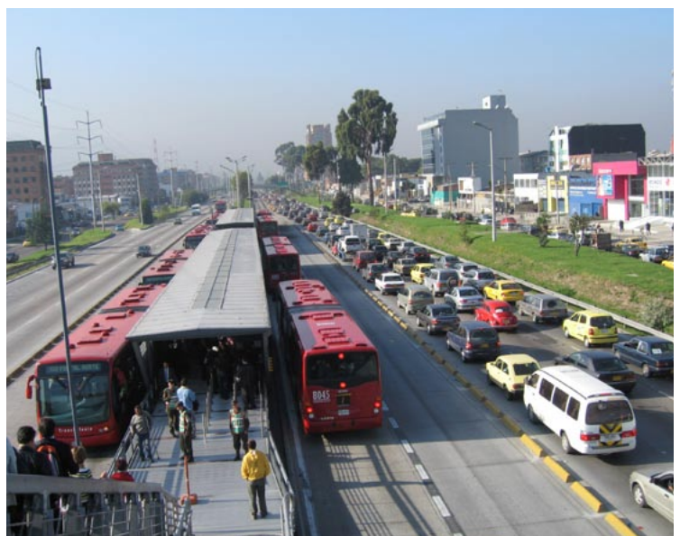
Figure 50 BRT stations are located on the median. Exclusive lanes ensure short travel times.
