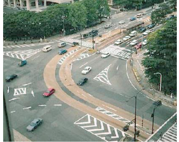
Fig. 9 Nagoya, Japan, marks the bus lanes with a coloured road surface. Courtesy of John Cracknell, TTC, and the US Transportation Research Board.
