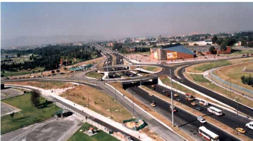
**Bogotá: North-South motorised traffic elevated, East-West motorised traffic depressed, and facilities for non-motorised travel are at ground level.**
