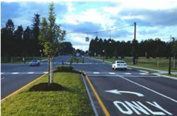
**After: The median on the far side is wider to reinforce the left turn lane. Note the bollards to protect pedestrians.**
