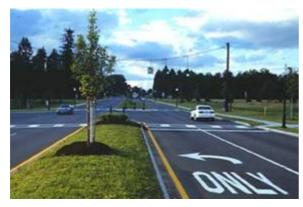
After: The median on the far side is wider to reinforce the left turn lane. Note the bollards to protect pedestrians. Reid Ewing
