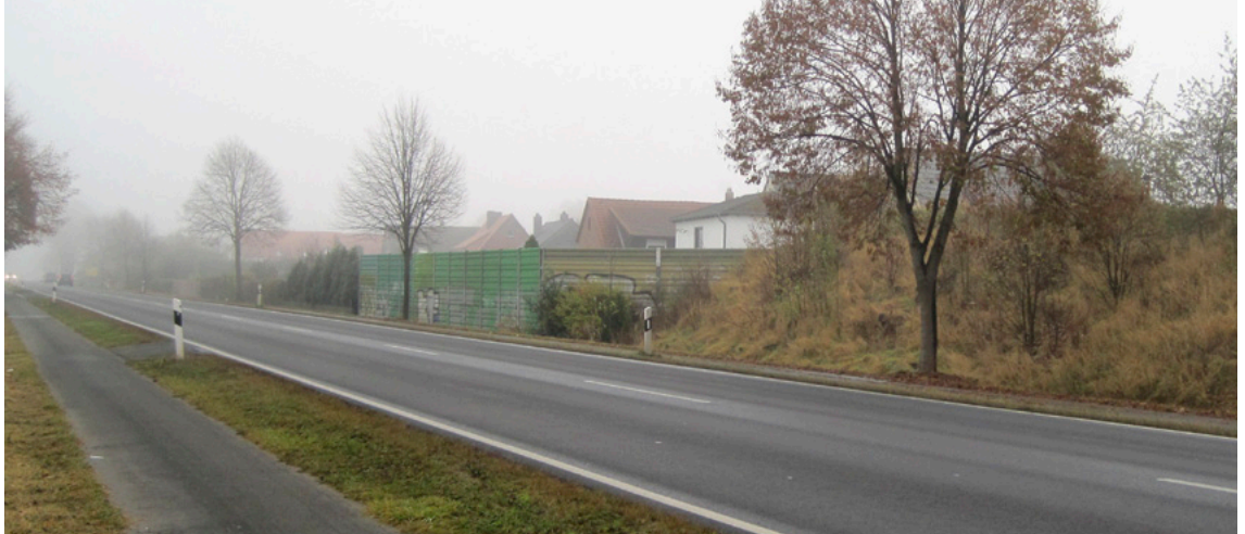
Fig. 22 Noise barriers designed as wooden or concrete walls (center of the photo) occupy less space than a heap-up earth wall (right side of the photo). Klaus Neumann, 2011
