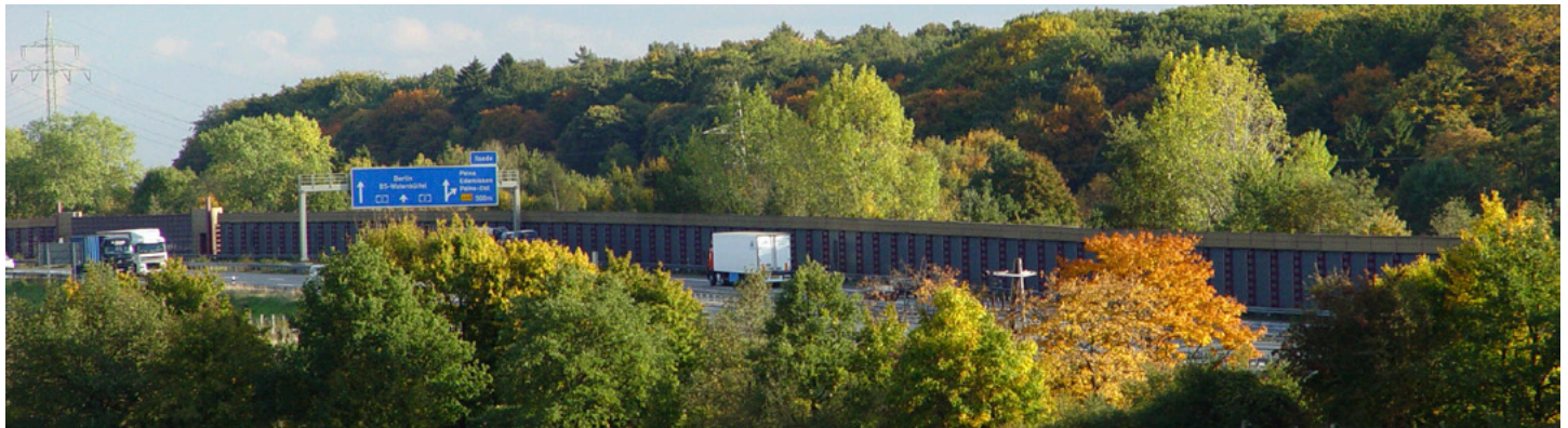
Fig. 23 A reasonable implanted noise barrier protects a near-by recreation-forest-area from the heavy noise emitted by the never-ending stream of cars and trucks on a highway in Germany. Klaus Neumann, 2009
