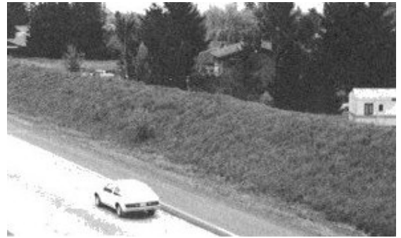
Earth Berm Noise Barrier
