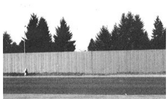
Concrete Noise Barrier with Woodgrain Texture
