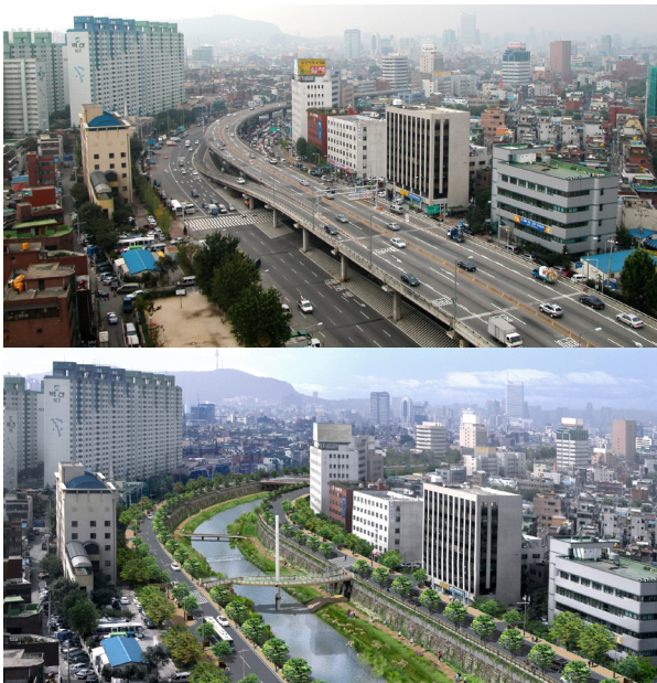
Figure 49. This restoration project in Seoul was carefully monitored, as these two photos of the same place along the Cheonggyecheon River show. Source: SDIK
