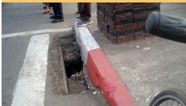
Figure 5: Hole at crossing on Tubman Boulevard in Monrovia. © Alexander Czeh
