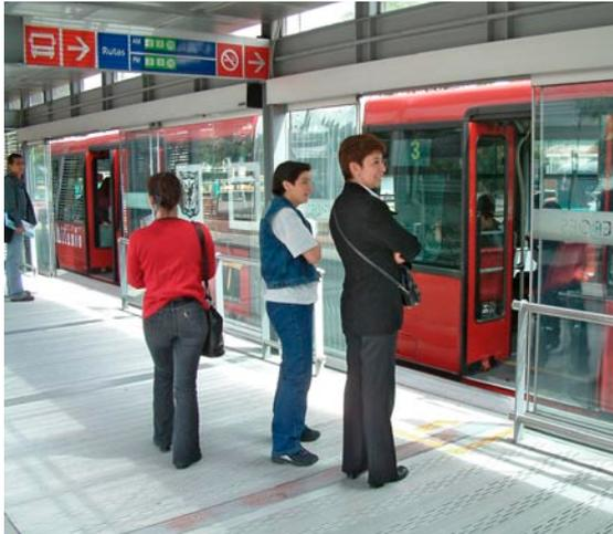
Bogotá has made use of sliding doors at the station to vehicle interface (Figure 53). Automatic station doors give a degree of safety to waiting passengers as well as protection against wind, rain and cold. Additionally, the sliding doors can help prevent fare evaders from entering the system. The disadvantage of the doors is that they are susceptible to mechanical failure and can thus add to system maintenance costs.
